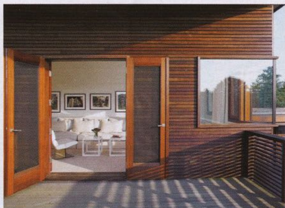
Walk The Line | An ipe rain screen cloaks an exterior volume of the main house, enclosing the kitchen on the ground level and guest accommodations (ABOVE) on the second. Three sides of glass form walls in the breakfast room (TOP), which resembles an outdoor pavilion punctuated by Ingo Maurer's dramatic Flotation light fixture. See Resources.
